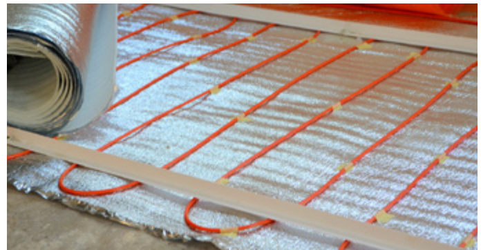
Underfloor heating provides consistent warmth around a shed.
