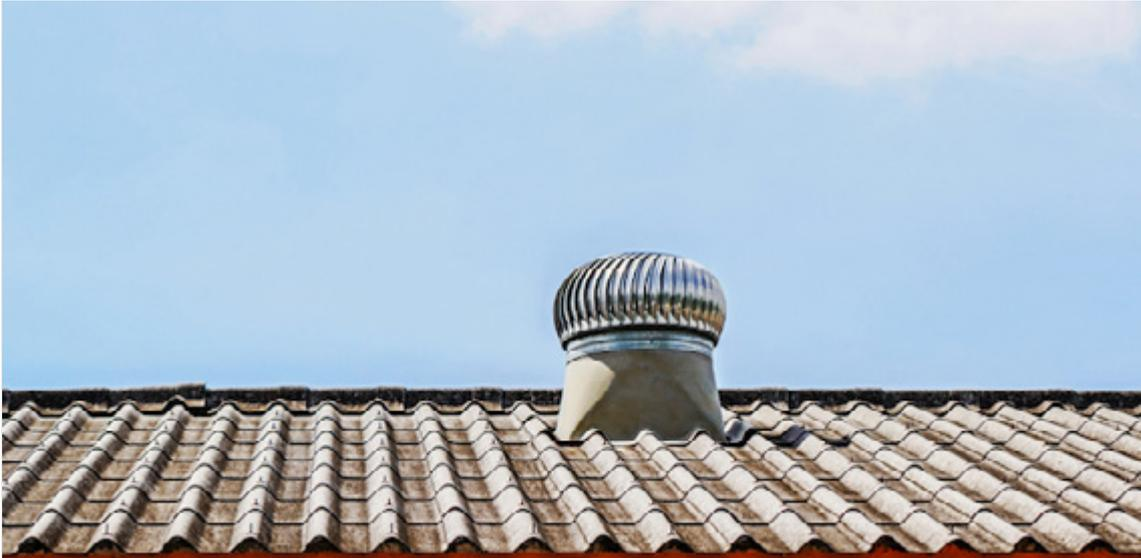
*This clever device uses wind power to draw hot air out of a building.*
