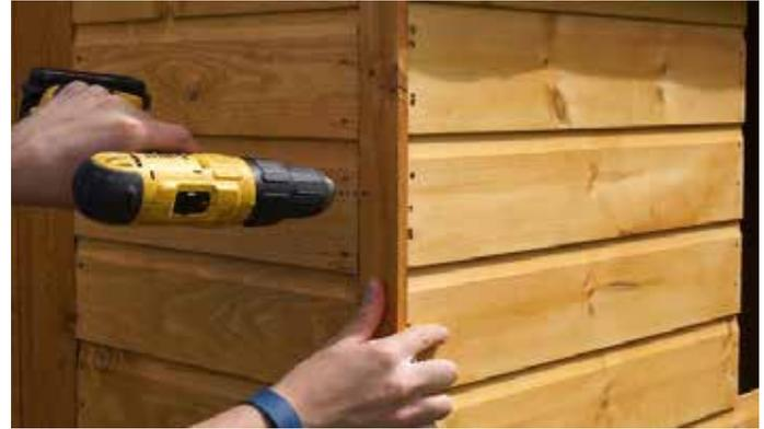
*Pre-drilling screw holes stops timber splitting.*
